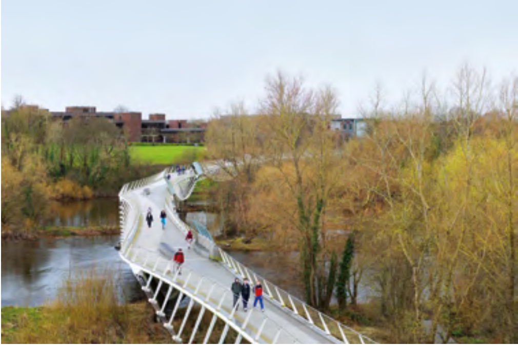
The Living Bridge connects the campus where the River Shannon runs through the University of Limerick.
