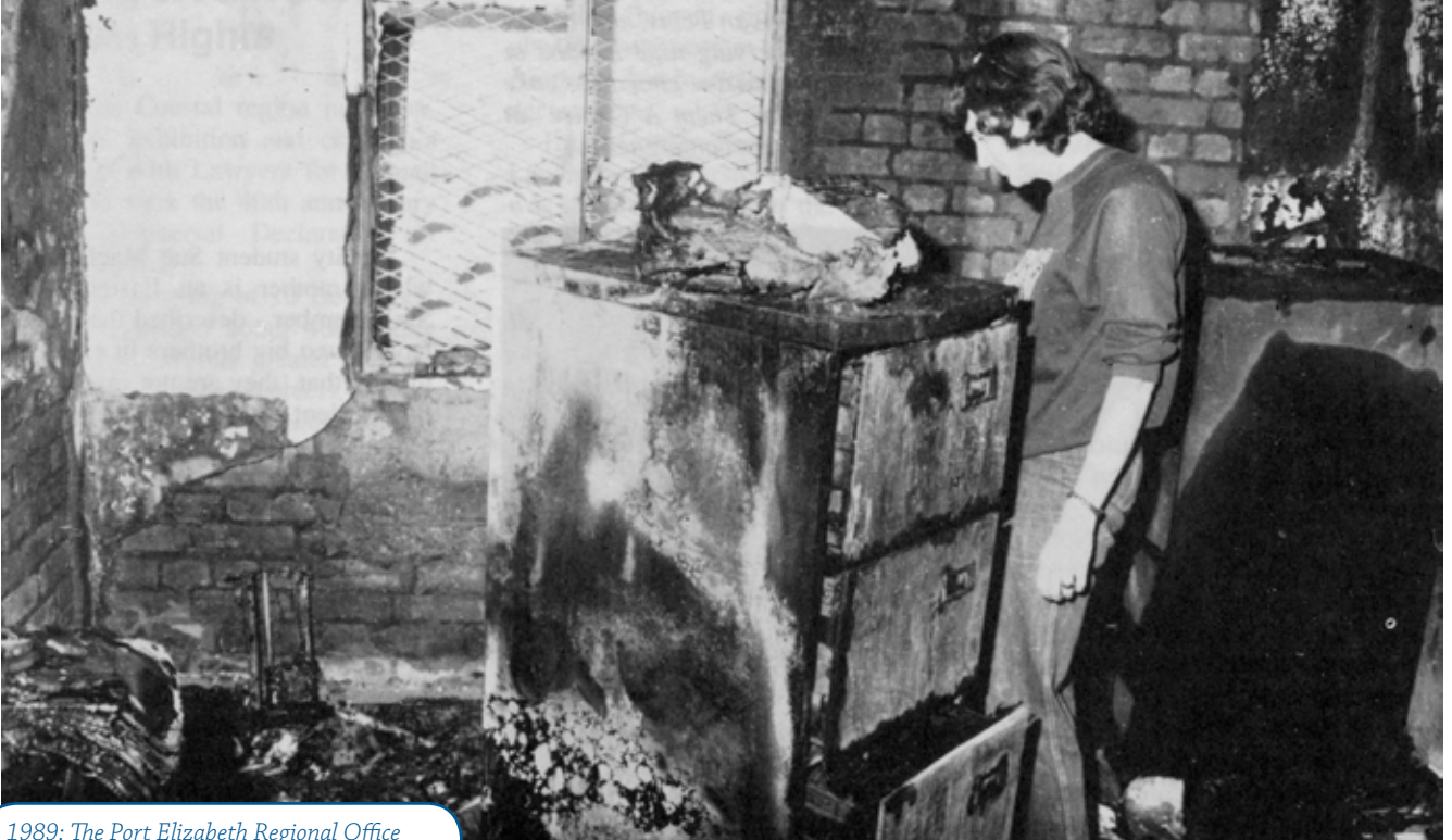
1989: The Port Elizabeth Regional Office was almost destroyed in an arson attack.
